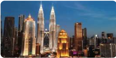
PETRONAS TWIN TOWER (SURIA KLCC)
